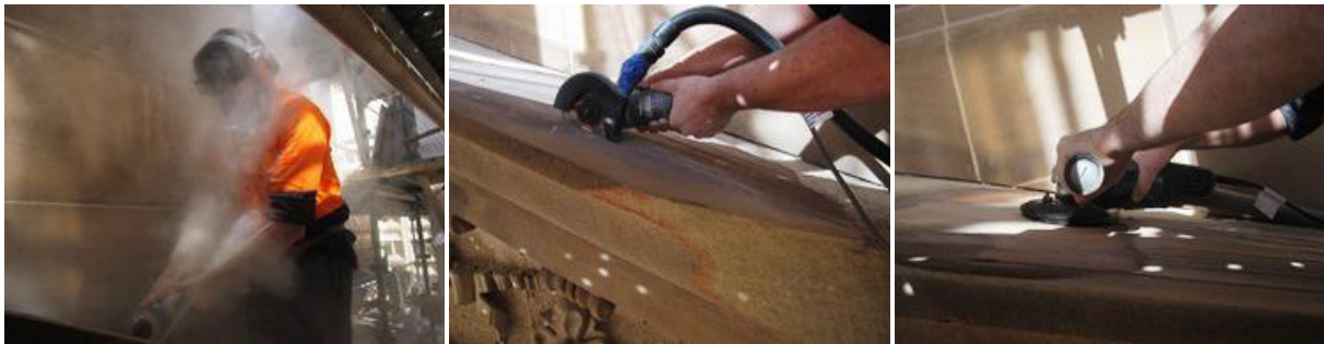
Figure 4: 'Chopping out' no dust shroud, Figure 5: 'Chopping out' with dust shroud, Figure 6: 'Spinning' with shroud Source K. Alamango 2015
