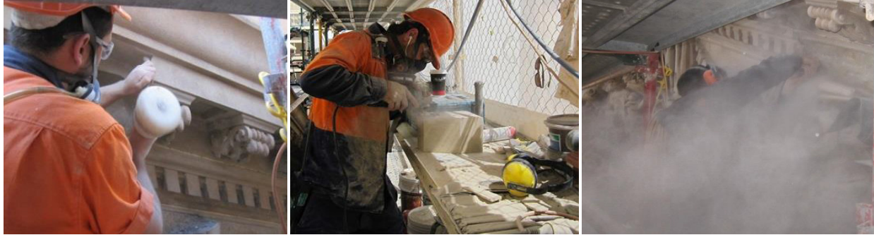
Figure 1: Lump hammer & chisel Figure 2: 'Spinning' with angle grinder Figure 3: 'Chopping out' with grinder
